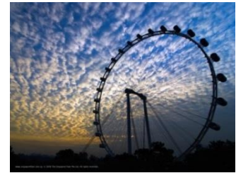
One A8n was installed at the ground level facing the wheel
