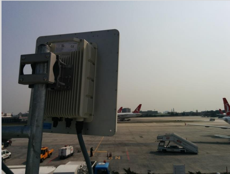
A8-Ein was installed for apron coverage
