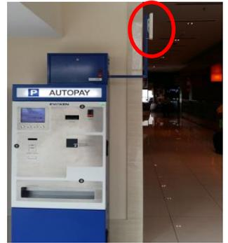
*The ticketing machine is connected with Altai C1n for wireless connectivity*
